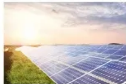
Energy Storage System
